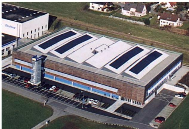
Technical data: 100 kWp monocrystalline PV power modules mounted on four shed roofs of 780 m<sup>2</sup> surface.
